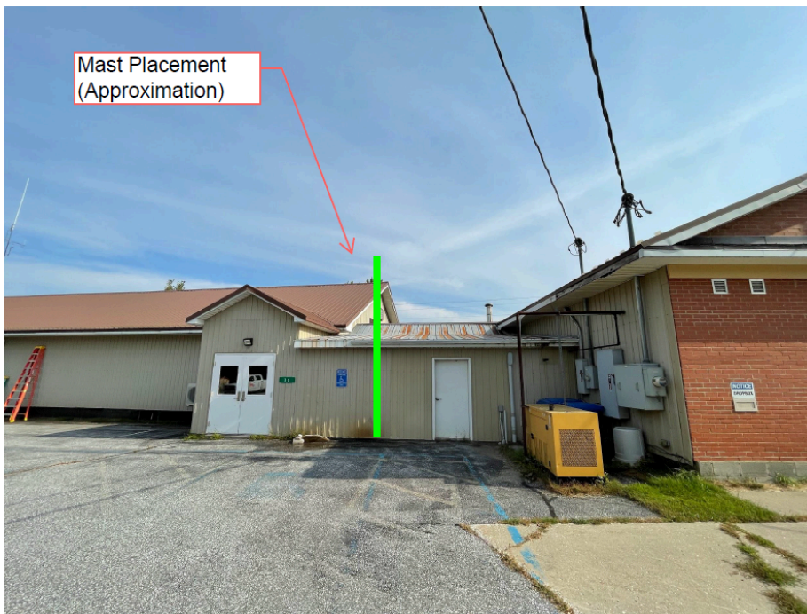
There will be two mast, one for Utility and one for Telecom use
